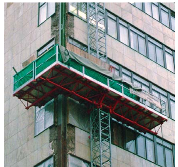
Platform can be turned 90° to the side of the main platform
